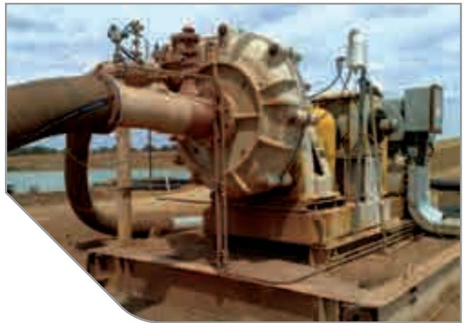
After installing AESSEAL® double seal and tank system
